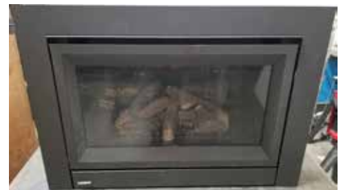
Completed Faceplate & Safety Screen Installation
